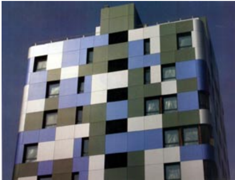
The rainscreen aluminium cladding on eleven new apartments by Arroyo and Gonzaga, in Oviedo, Northern Spain, proclaim their freedom from sense with 'dithered' window-placings as well as a 3-colour "pixel blur". The effect destroys reason.
